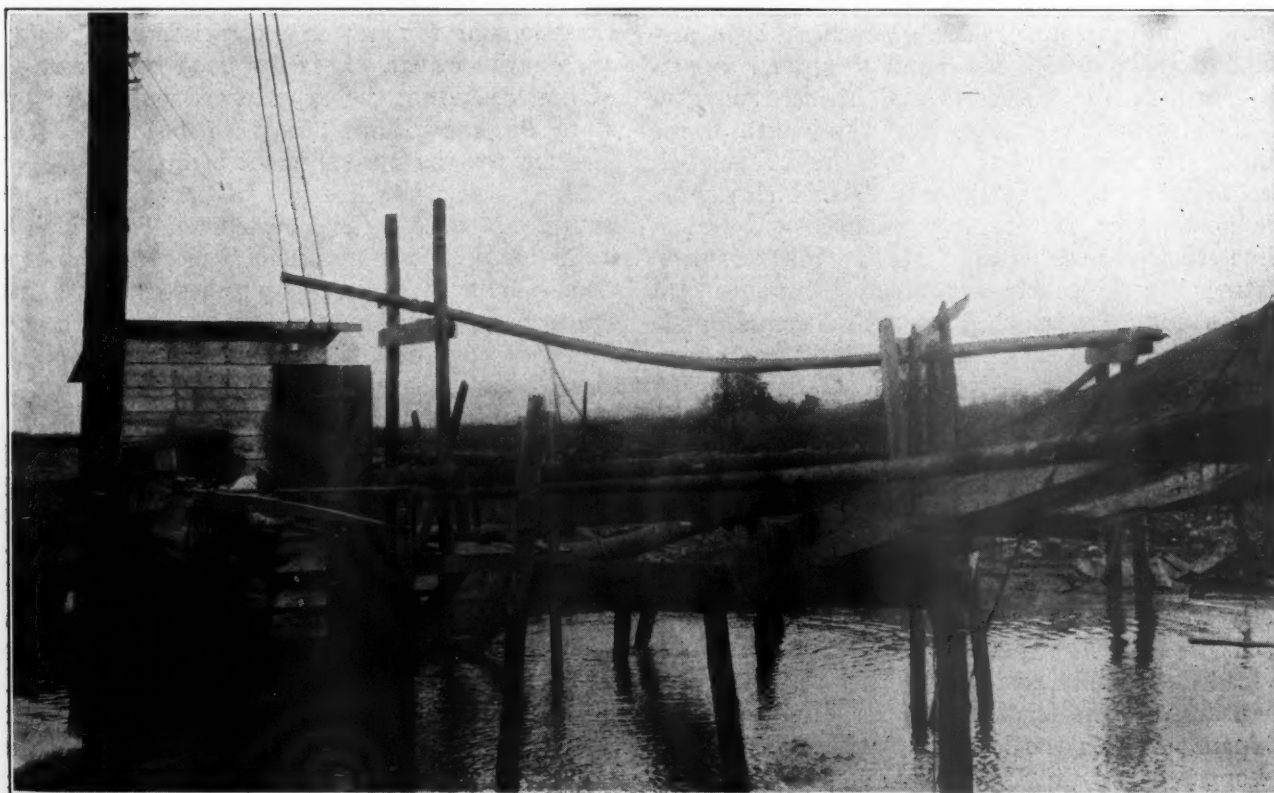
A View of the Sump
